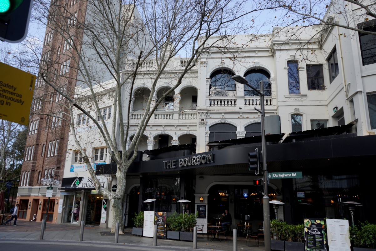
Figure 6: The facade of The Bourbon at 22-24 Darlinghurst Road, Potts Point
